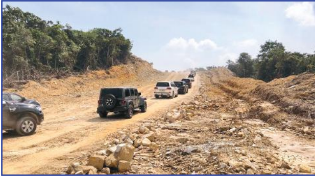
The condition of the road after rock breaking and clearing
